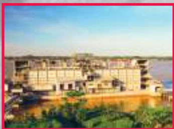
9 Terminal Palaran Samarinda, Kalimantan Timur Palaran Terminal Samarinda, East Kalimantan
