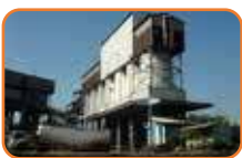
Land Cement Silo Cigading Serang, Banten Cigading Cement Silo Serang, Banten
